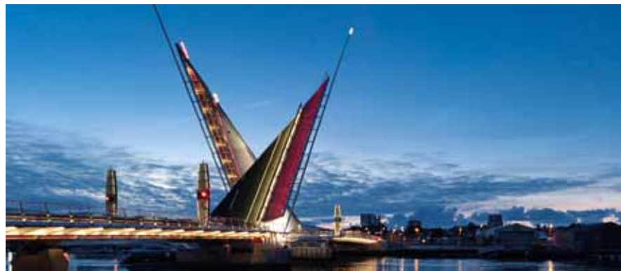
Fot. 1. The Twin Sails Bridge, Poole, Wielka Brytania ( www.steelconstruction.info )
