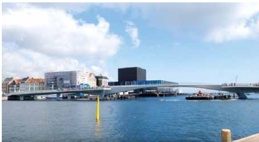
Fot. 2. Inner Harbour Bridge, Kopenhaga, Dania ( www.e-architect.co.uk )
