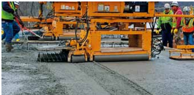
5. Eisenhower Memorial Bridge w Red Wing.
